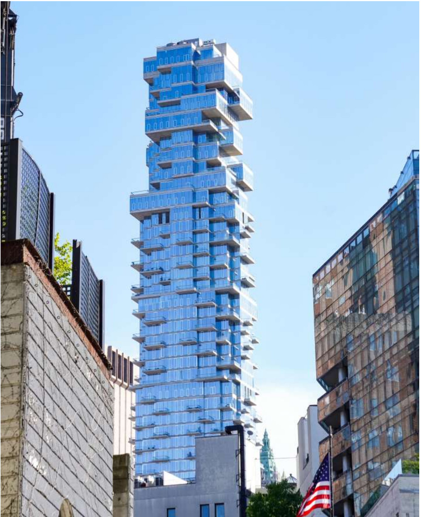
Material Supplied - Jenga Tower, Manhattan NY
